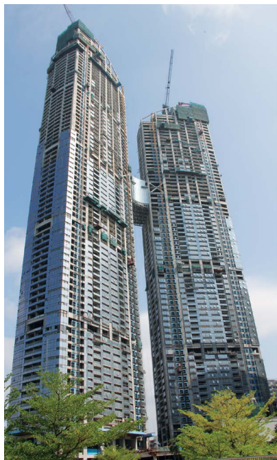
The team led by Felix worked out a reinforced concrete structure underpinning the two 300m residential towers of the East Pacific project.
