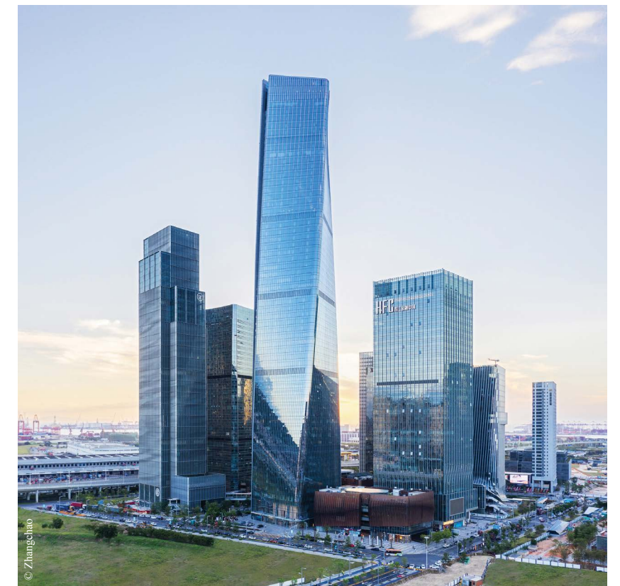
Shimao Qianhai Centre is the tallest twisted building in China. The team led by Felix developed an innovative twisted frame-core wall structure system to realise the building's unique spiral shape.
